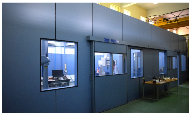
Fig. I.3.2: Outside view of the enclosure in Metrology Hall.
