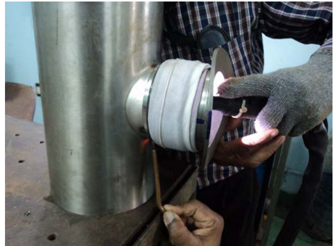
Fig. A.9.2: GTAW of transition piece with 2 phase pipe.
