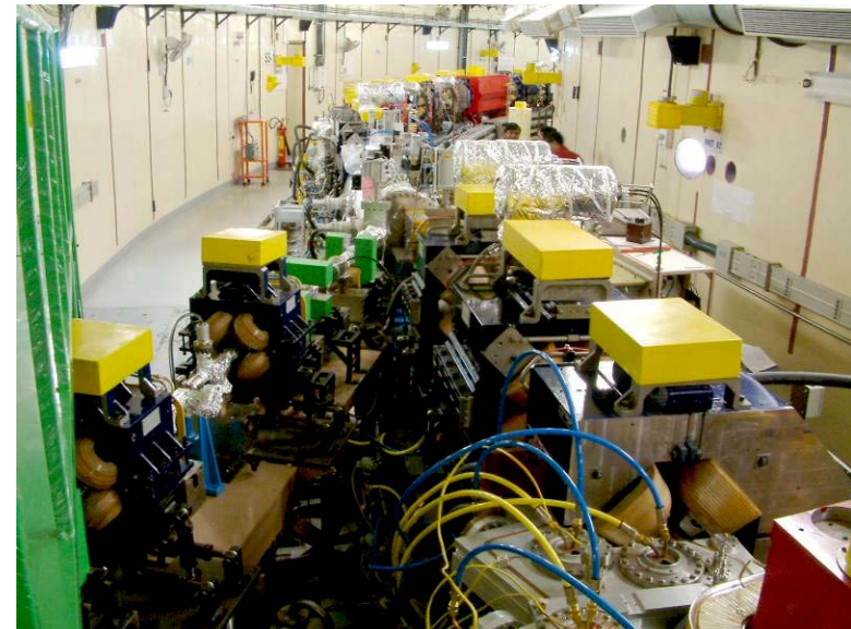
Transport Line-3 Joining on to Indus-2
