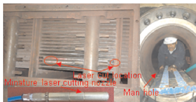
Fig. L.2.2: Actual laser cutting location in SG of KKNPP-2 with man hole and laser cutting nozzle.
