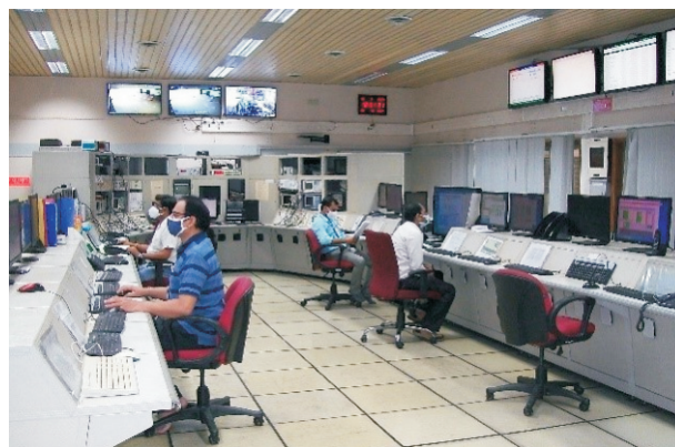
Fig. A.1.4: A view of Indus control room depicting work environment complying with COVID-19 related guidelines.
