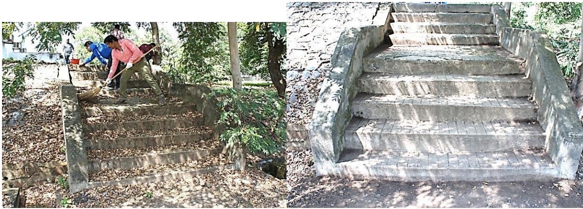
ADL Staircase towards IMA building
