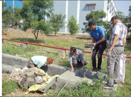
Cleaning the choked drainage trench (South side of the building)
