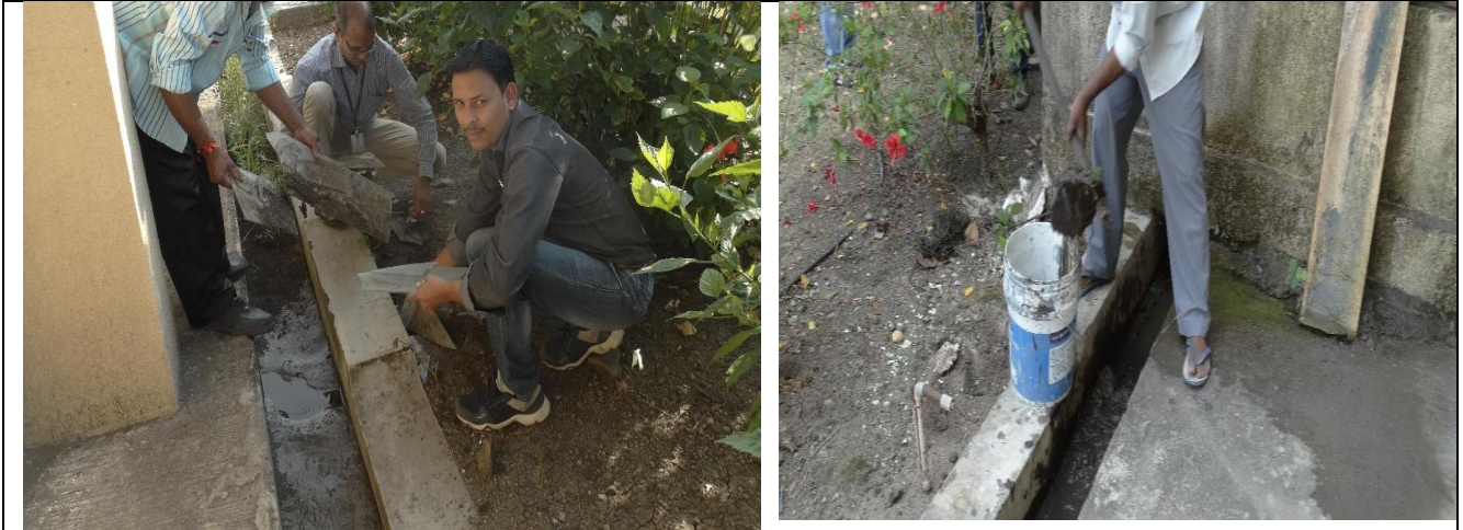
Cleaning of drainage near walls of R&D Block G building
