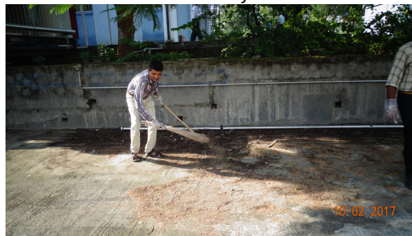
Outside R&D Block-A during the SEVA
