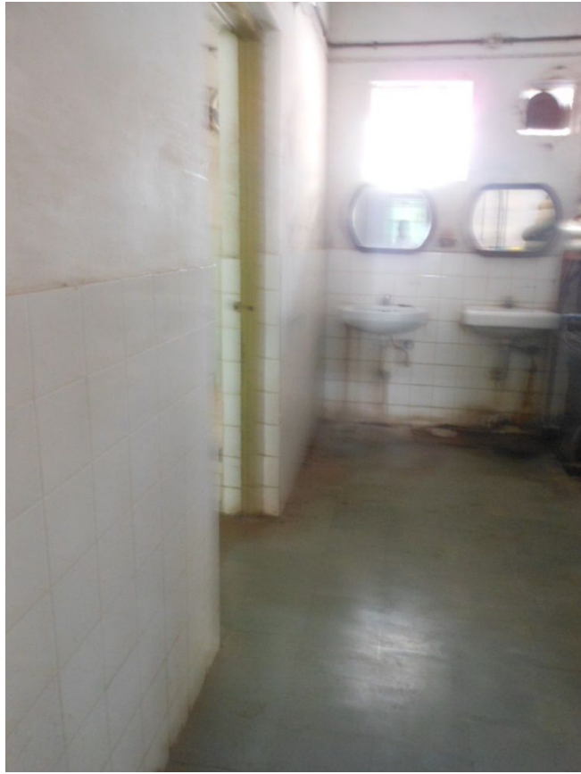
LCW Plant Building-Toilet Area
