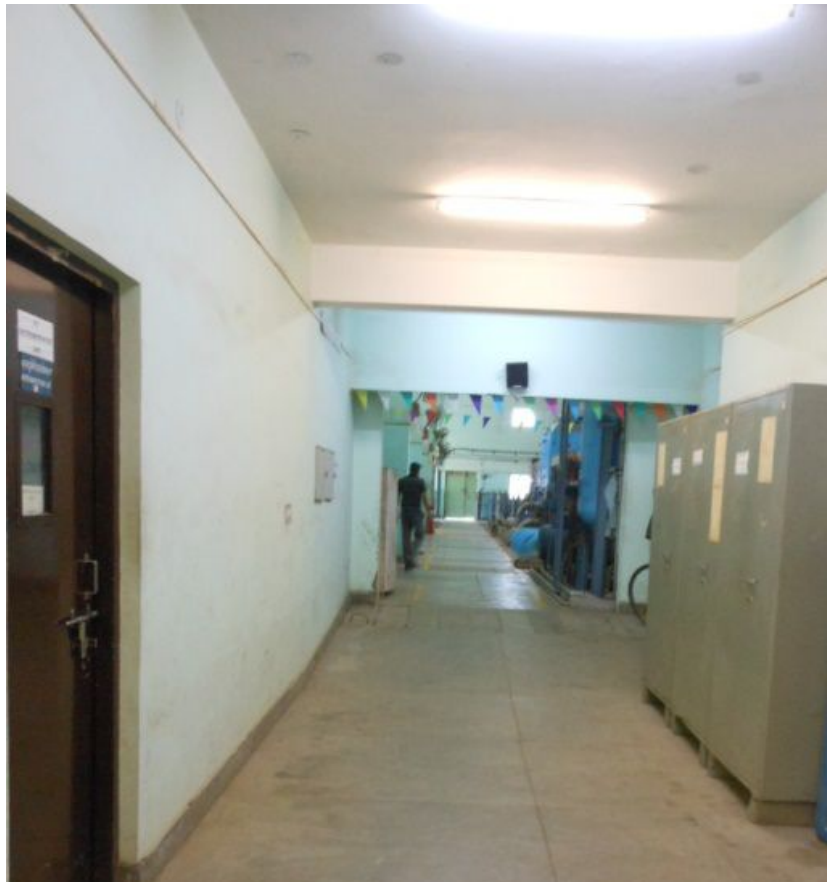
LCW Plant Building- Working Area
