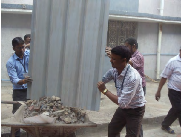
Collecting the building construction waste material
