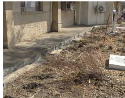
After cleaning near back wall of Block G
