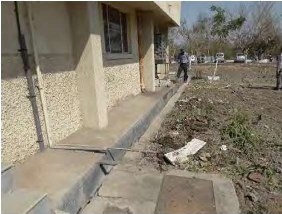
Before cleaning near side wall of Block G
