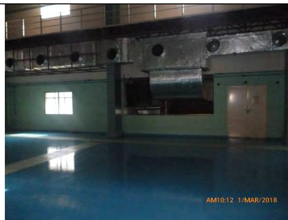
H- building main Hall (After)
