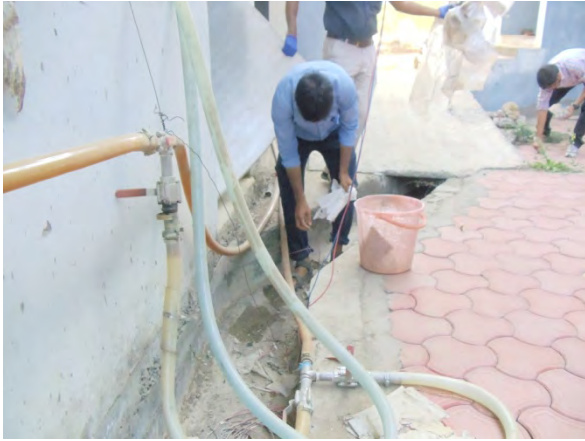
Trench cleaning SCRF building back side
