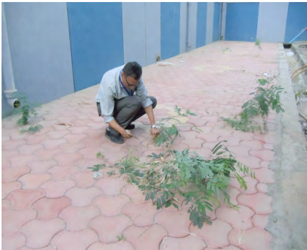
SCRF Building back side Lawn area before
