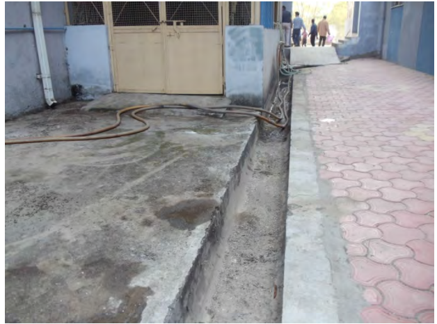
Trench after cleanliness drive
