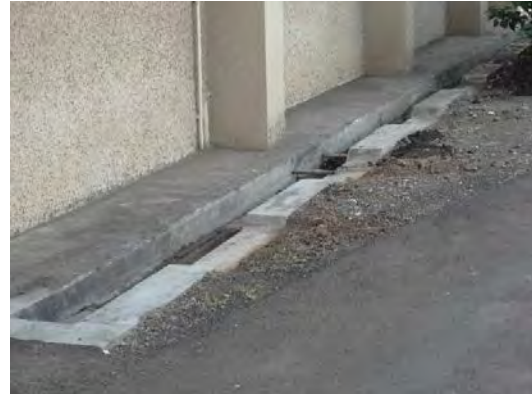
After cleaning outside front wall of Block G
