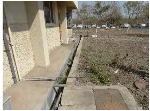
After cleaning near back wall of Block G
