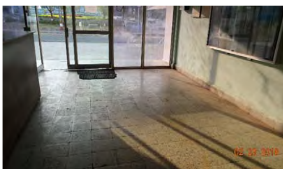
Entrance of R&D Block-A after the drive
