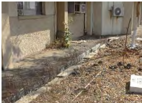
Before cleaning near back wall of Block G
