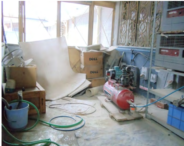
EBW Chiller Shed Before (SCRF Building)
