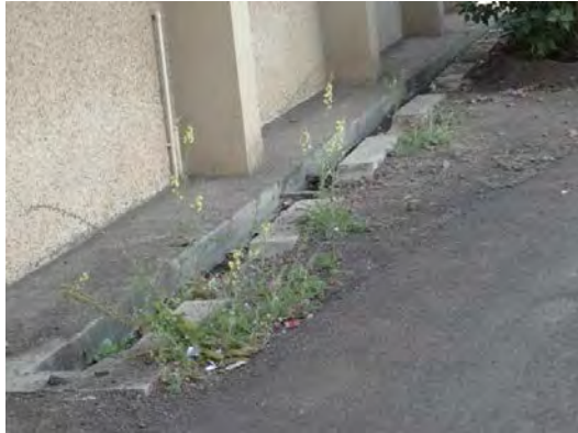
Before cleaning outside front wall of Block G
