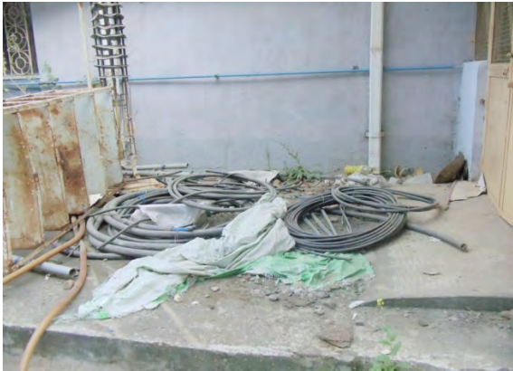
SCRF Building back side area before
