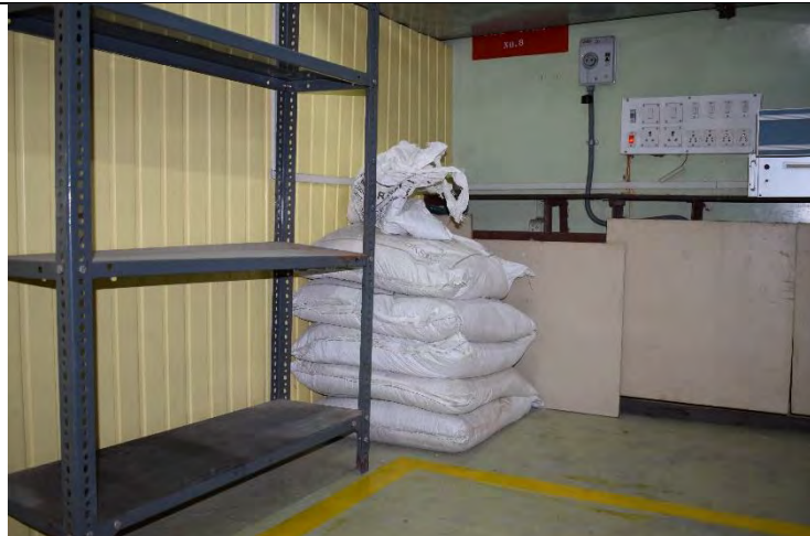
LPSD: D 6BLOCK, ROOM NO. 117, LASER POWER SUPPLY HALL (PARTITION-2)
