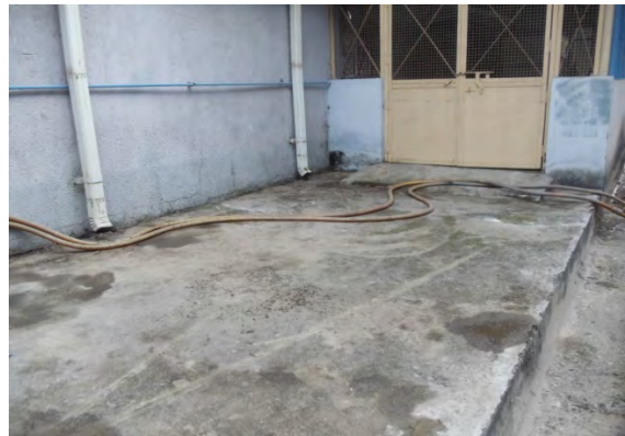
SCRF Bld back side area after cleanliness drive
