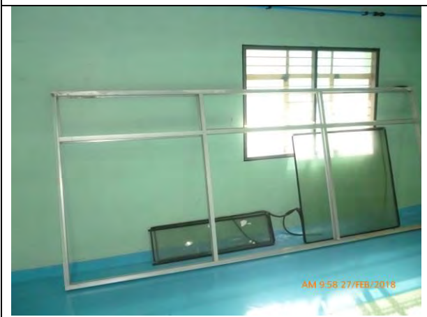
H- building main Hall (Before)
